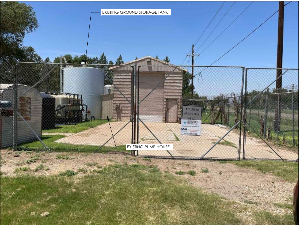
TOWN NORTH ESTATES PUMP STATION SITE
